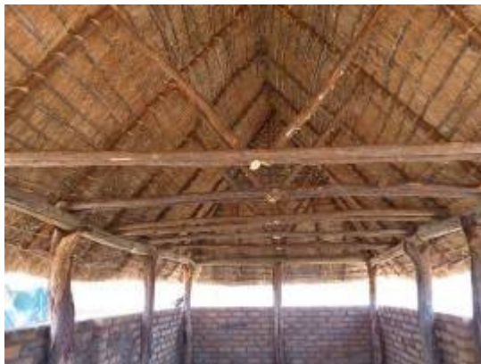
A typical grass roof construction
