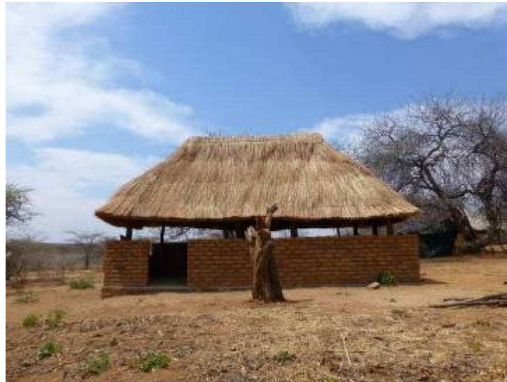
The newest of our bandas, constructed with bricks made locally from soil, water and the heat of the sun
